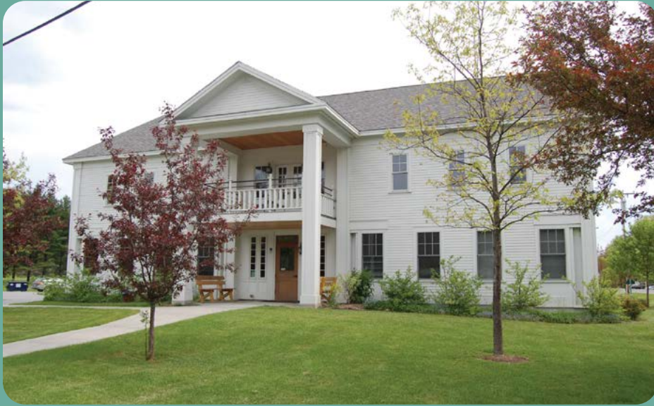
869 Old County Road Waitsfield, VT
